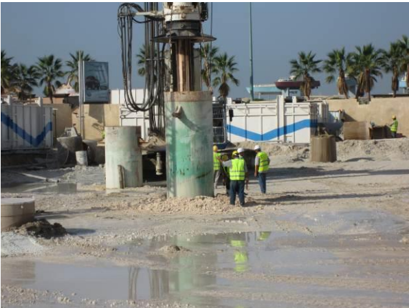
Figure 13 Installation of the casing
