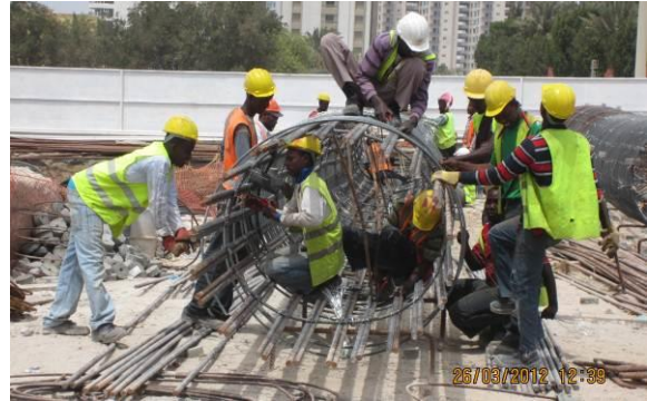
Figure 14 Construction of Reinforcement Cages
