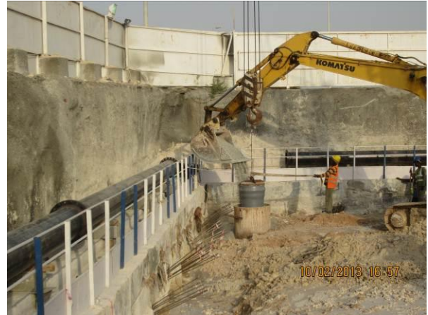
Figure 22 Installation of the Gravel Filter at a Well
