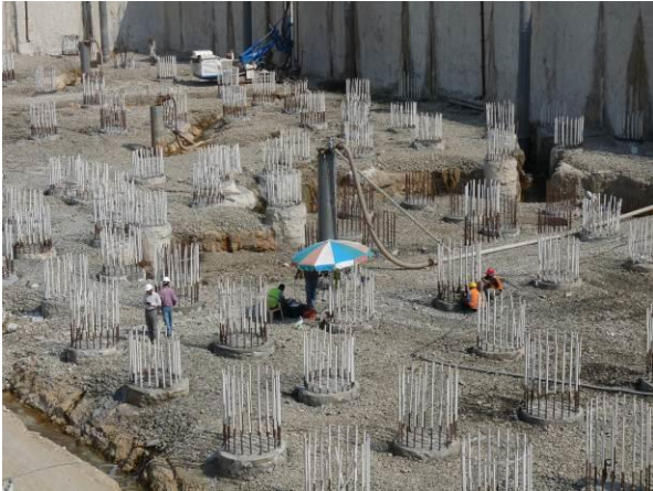
Figure 16 Bore Piles in the Area of the High-rise foundation
