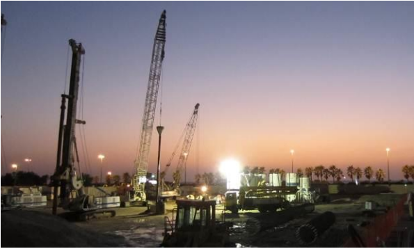
Figure 12 Pile Construction, Drilling Work
