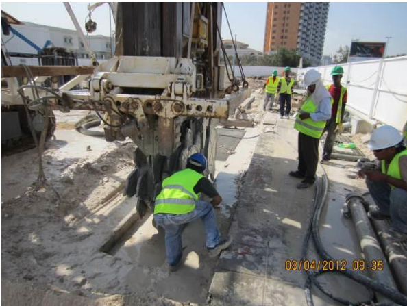
Figure 17 Construction of the Diaphragm Wall
