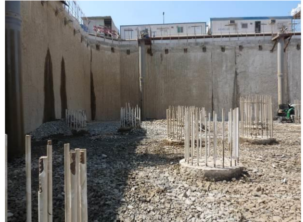
Figure 18 Diaphragm Wall during Excavation
