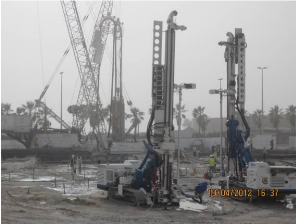
Figure 20 Drilling Equipment for Injection Boreholes
