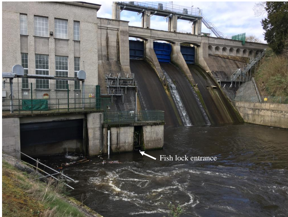
Figure 5. The first Borland fish lock at Leixlip Dam (Photo: Redeker)
