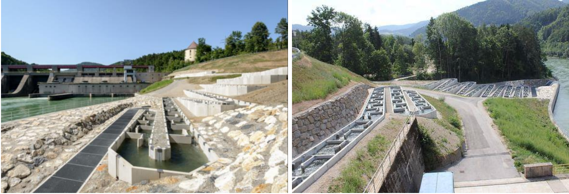
Figure 4. Enature Fishpass at Schwabeck Hydropower Station, Drau River, Austria. Designed for coarse species: 158 pools (LxW = 3.0 x 2.17 m), slot 0.4 m wide, max. 0.13 m drop per pool, discharge = 0.45 m 3 /s (Photos: Verbund).
