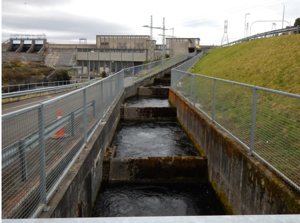
Figure 1. Pool & traverse fish pass (72 pools, 28.5 m head) at Cathleen's Fall Hydropower Station, River Erne, Ireland. Designed and built for Salmon in the 1940's, with each pool 7.62 m long by 3.66 m wide with a 0.46 m drop between each pool. (Photo: Redeker)
