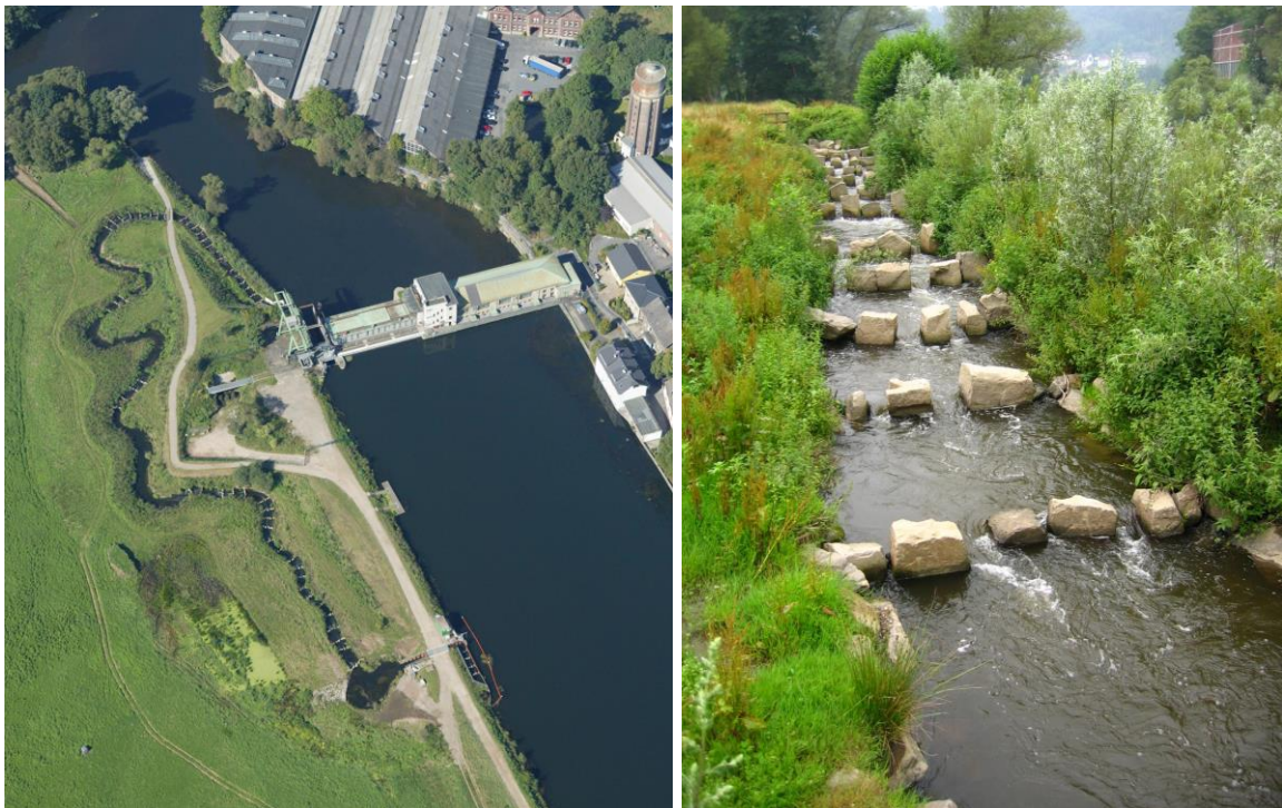
Figure 3. Nature-like bypass channel at Harkortsee Hydropower Station, Ruhr River, Germany. Left: Aerial view (Photo: Ruhrverband); Right: Pool section (Photo: Redeker). Designed for course species: Total length = 375 m, 57 pools, 2 slots per boulder row ~0.35 m wide, max. 0.13 m drop per pool, discharge = 0.7 m 3 /s plus 0.5 m 3 /s auxiliary flow.
